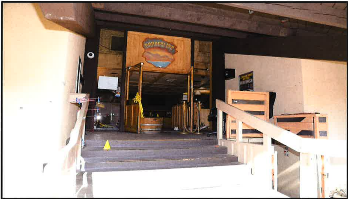
Front porch of Borderline; photo shows trajectory rods in the left (west) handrail. The surveillance camera (CAM 9) can also be seen in the upper lefthand corner.
