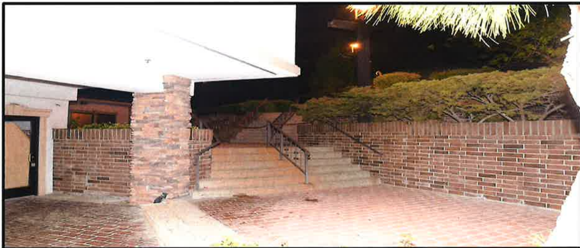
Photo depicts south side of the Borderline bar; illustrates the elevation difference and the concrete stairs that lead up to the walkway/sidewalk outside the bar.
