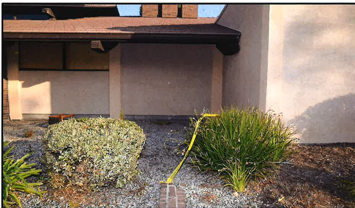
Glass windows on the south side of Borderline Bar and Grill (east of the brick fireplace). Opposite the right (or east-most) window is where the DJ booth is located.
